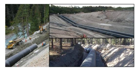
Buried gravity pipes are evaluated for suitability by demonstrating that the stresses due to burial loads can be safely accommodated by the pipe. The design methodology for burial assessment is well described in various plastic pipe handbooks, and the National Bridge codes (AASHTO and Canada).
